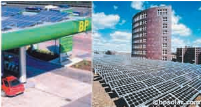
BP service stations (left) can be fitted with solar systems capable of providing power for pumps and canopy lighting.
