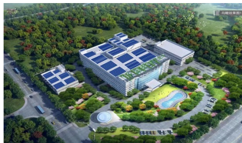
Figure XX Aerial view of Phase I of Suzhou Gold Project
