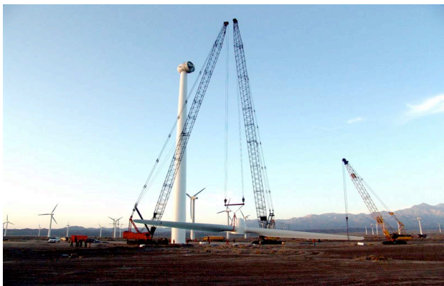
Installation of China's first domestically manufactured MW-scale wind turbines at Dabancheng Wind Farm
