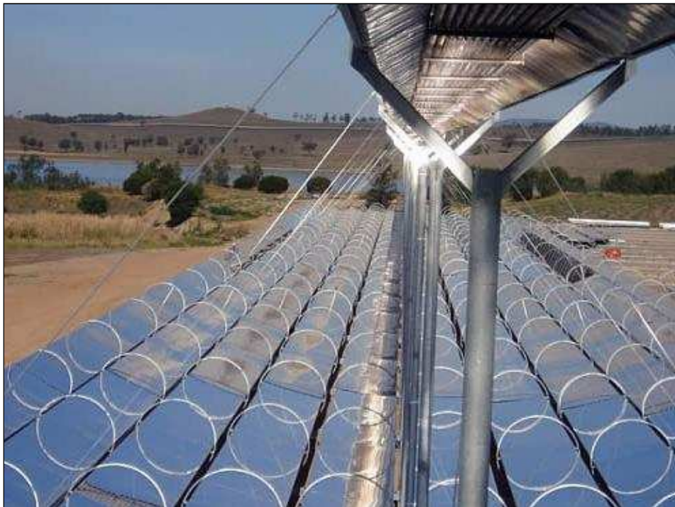
Figure 2-8: Fresnel reflectors of a LFR power plant /Greenpacks 2008/
