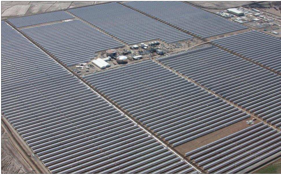
Figure 3-5: Parabolic trough power plant Andasol 1 /SM 2008/
