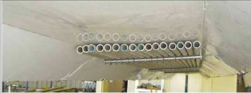
Figure 2-9: Absorbers of a LFR power plant /Pye 2008/
